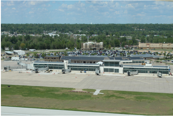
Source: Quad Cities International Airport
