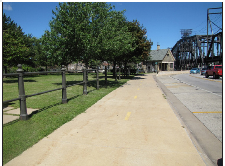
Figure 2.4 – Mississippi River Trail and Fort Armstrong Avenue, Rock Island Arsenal at Government Bridge
