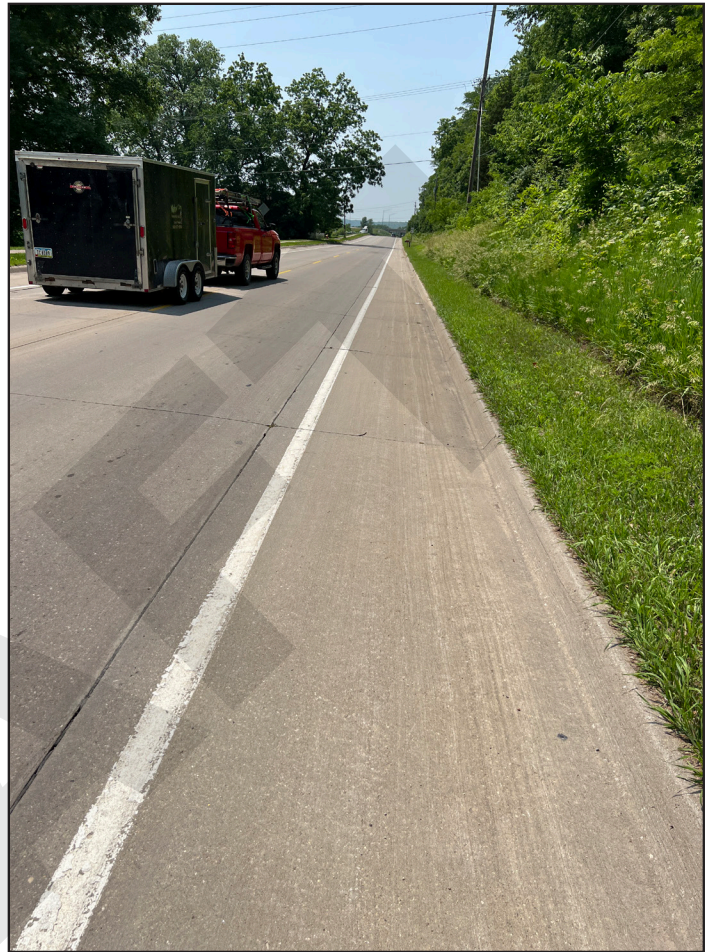
A shared roadway with a paved shoulder (No Bikeway Designation) in Muscatine County
