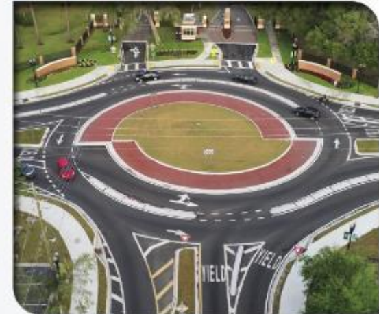
Source: Turbo Roundabout (Jacksonville, Florida), FHWA
