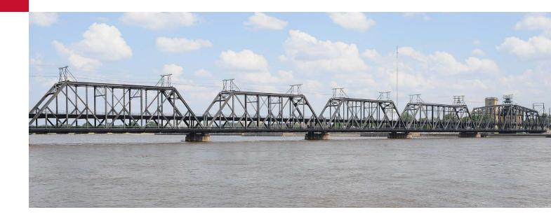
The Government Bridge is a twin-deck structure that accommodates the IAIS rail traffic on the upper deck and vehicle and pedestrian traffic on the lower deck. The roadway portion on the bridge consists of a two-lane public roadway with sidewalks on either side. A vertical clearance of 11'-8" and horizontal geometry at the lowa approach to the bridge restrict the type of trucks that the bridge can accommodate.
